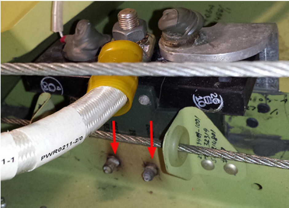
Figure 6. Internal Electrical Damage
